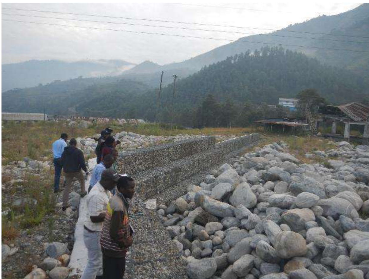
Photo 8-1: Gabion walls used to stabilise the river and protect the banks
