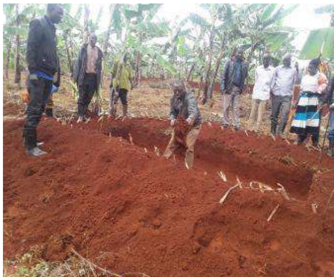
Figure 8-5: Infiltration trenches/ pits
