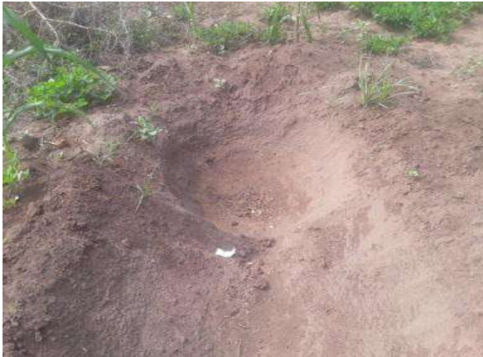
Figure 8-6: Cut-off drains and percolation pits
