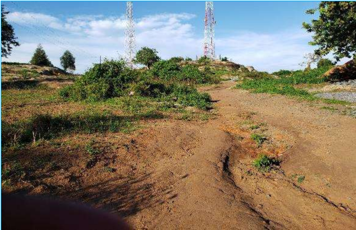
Figure 3-12: Access Road to reservoir site in Kidera RGC
