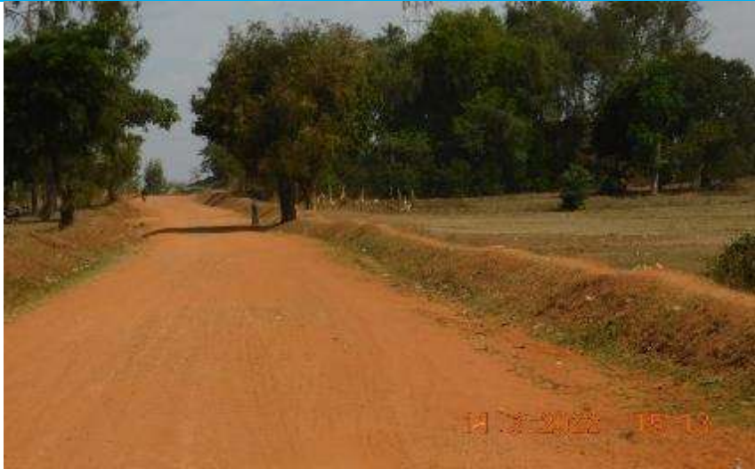
Kabugudho Road crossing
