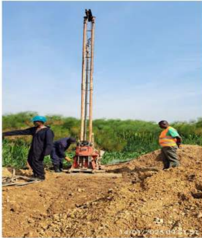
Figure 2: Bore hole drilling at the masindi port
