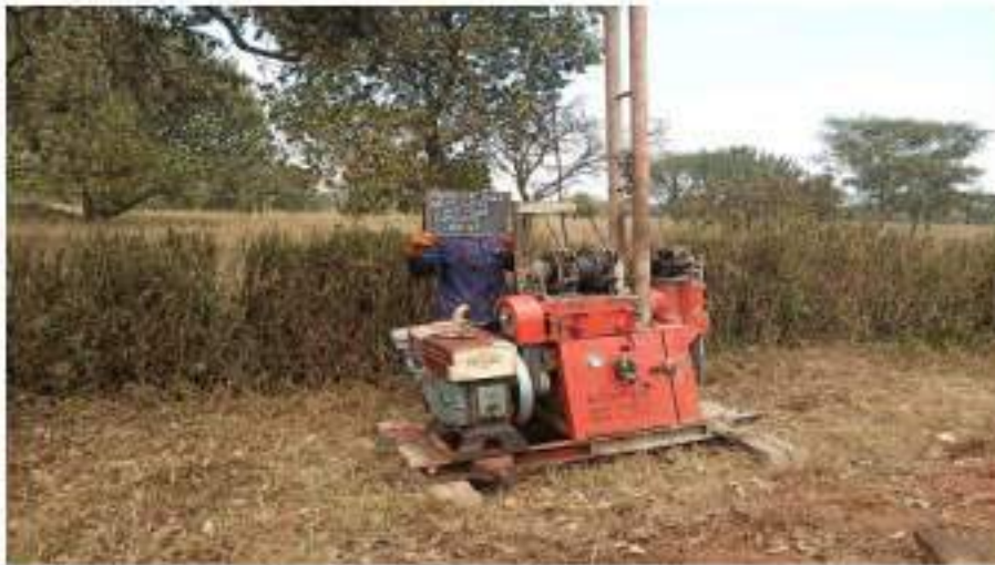
Figure 11: Drilling along the proposed alignment
