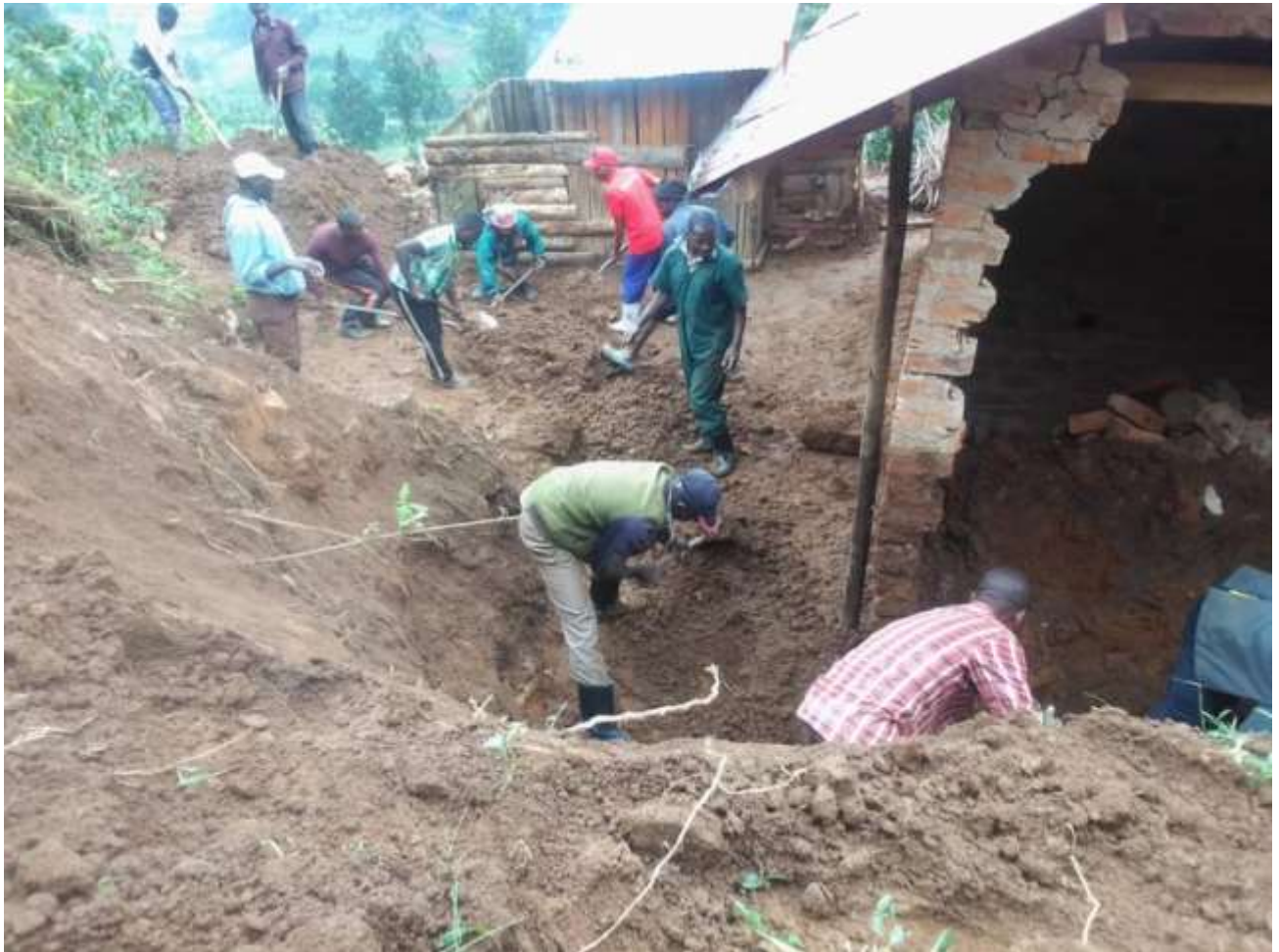
Figure 32: Shows the community members digging out the Landslides buried homes in Kisoro, Uganda, September 2022. (Uganda Red Cross)
