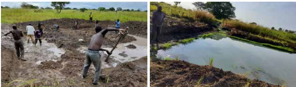
Figure 17: On the left; a water harvesting pond under construction in Alebtong district Gegere Subcounty and on the right; a fully constructed water harvesting pond with stabilized bunds and fenced with milk tree.
