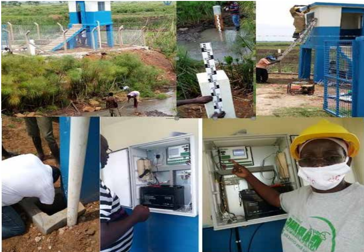
Figure 20: Digital water level monitoring station installed at Aleres in Pallisa district
