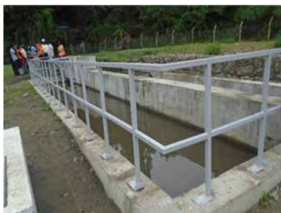
Figure 66: Intake chambers at Rwengaaaju Irrigation scheme in Kabarole District
