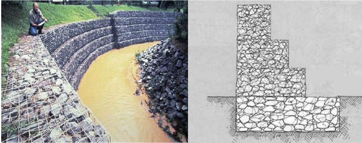
Figure 2 - Sample of Gabion layout
