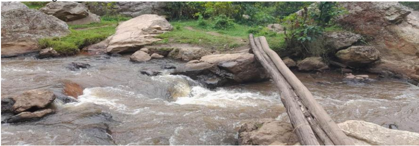
Plate 17: The existing temporary bridge made of poles to ease crossing near the proposed intake on River Kitakure
