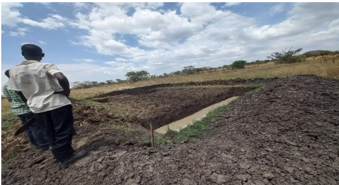
Plate 8: Fish Pond being excavated along the inlet to the dam
