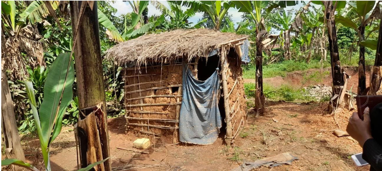
Plate 15: The type of the pit latrines within the project area of Igayaza
