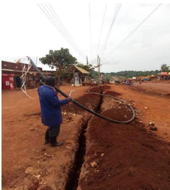
Extension of water in Mabaale town
