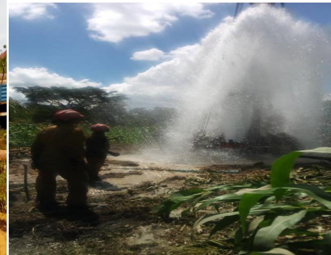
Drilling of a production borehole in Bukuya town, Mubende district in order to boost water supply in the area
