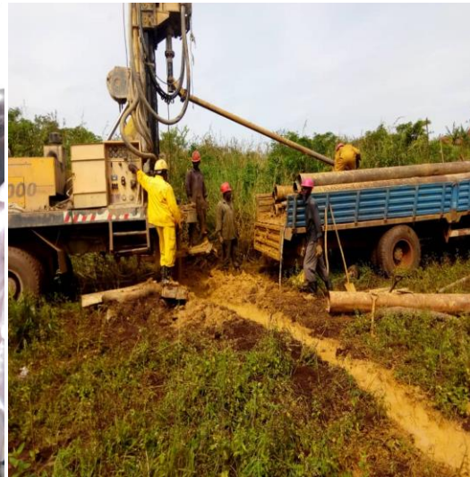
Drilling of a production borehole in Bukuya town, Mubende district in order to boost water supply in the area
