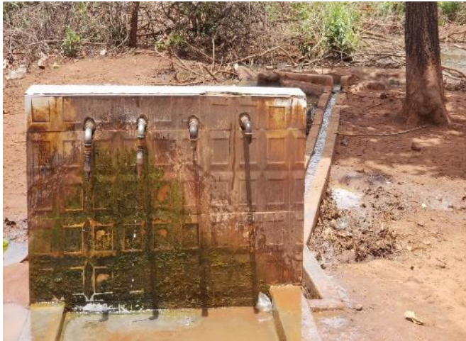
Piped water in Agoromin City Kitgum District
