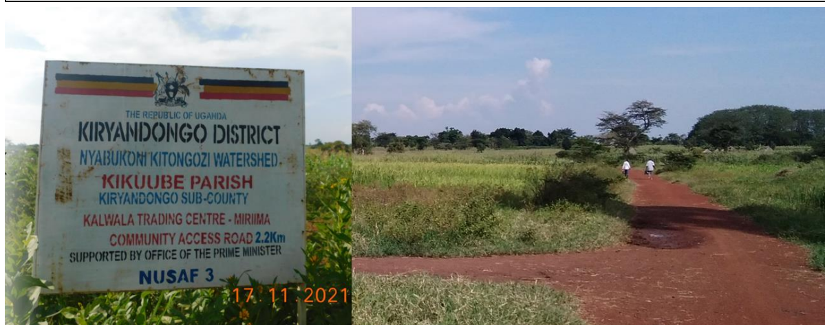
Figure 5-76: Kalwala – Mirima Community Access road
