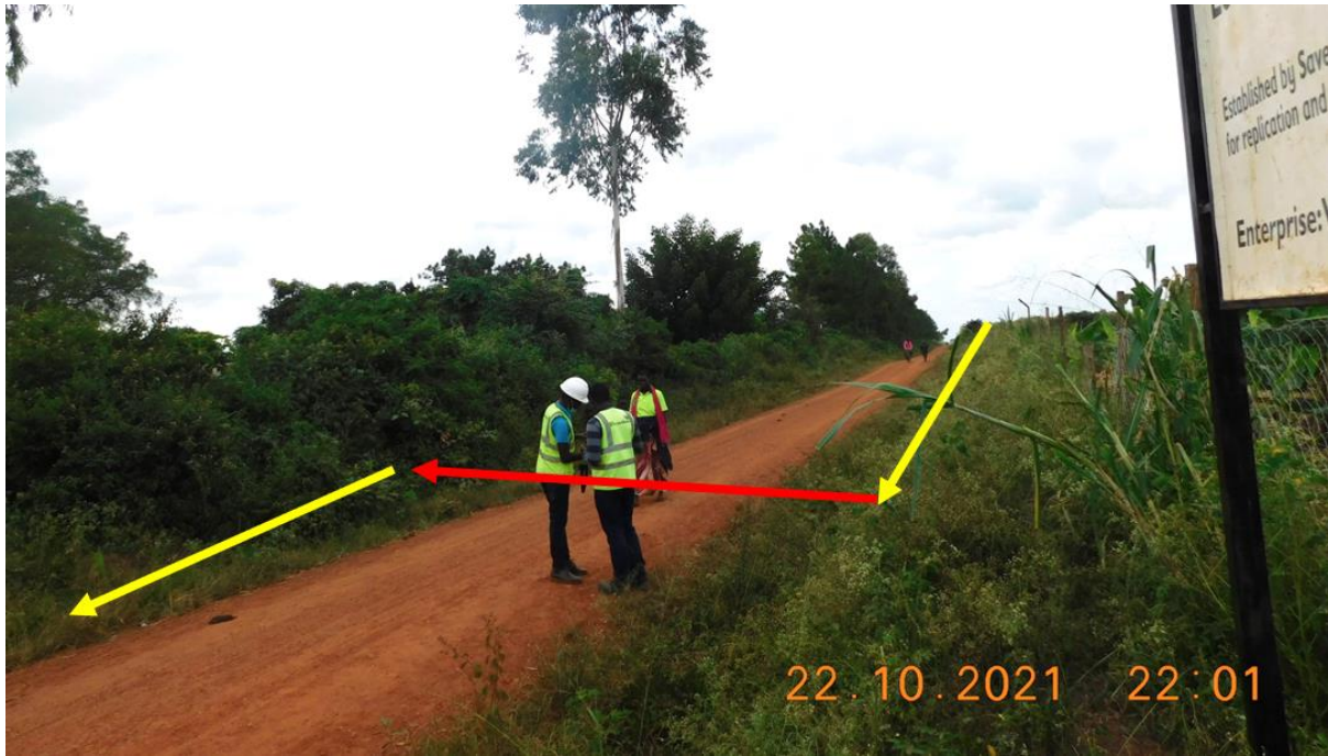
Figure 5-11: Transmission lines crossing the access road crossing at E408034, N209256
