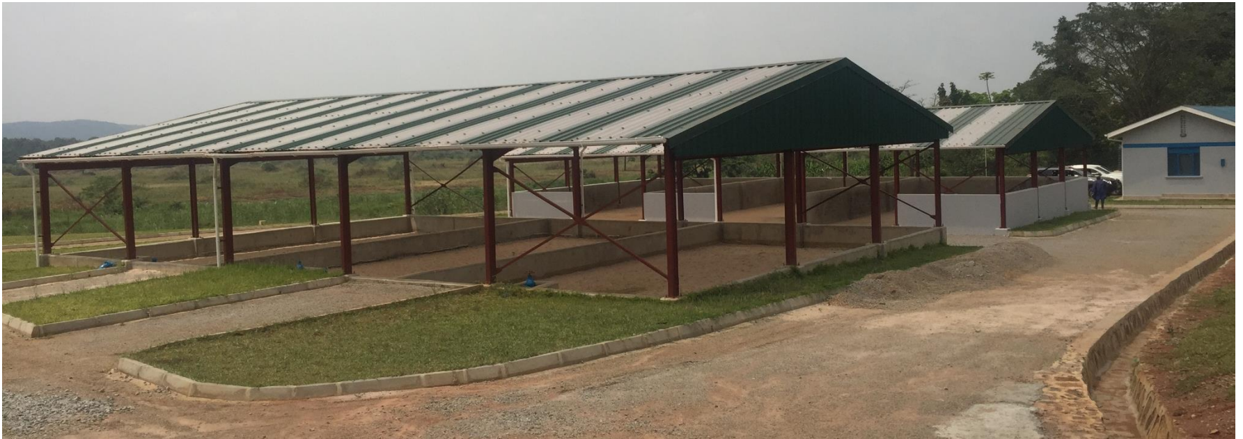
Newly completed FSTP in Kiboga town
