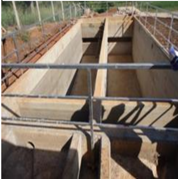
L-R: Thickening/settling tank; anaerobic buffer load reactor; and facultative ponds of Kiboga faecal sludge in Kiboga district.
