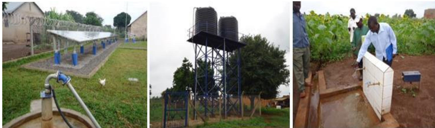
L-R: A water source and solar array; reservoir tanks; and community PSP of Kalwala mini solar powered scheme in Kiryandongo district.
