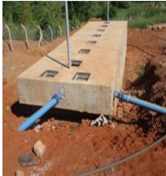
L-R: Thickening/settling tank; anaerobic buffer load reactor; and facultative ponds of Kiboga faecal sludge in Kiboga district.
