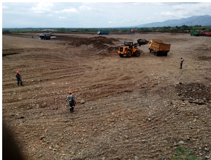
Ongoing excavation work for dam construction at Mubuku II Irrigation Scheme in Kasese District
