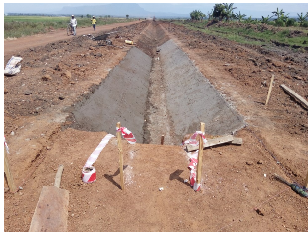
Irrigation canal under construction at Dobo II Irrigation Scheme to increase agricultural productivity, Butaleja District.
