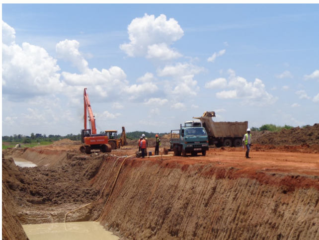
Excavation of main canal at Tochi Irrigation Scheme in Oyam District.
