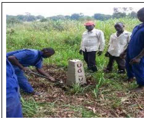
Figure 9.1 A pillar being planted at a wetland boundary
