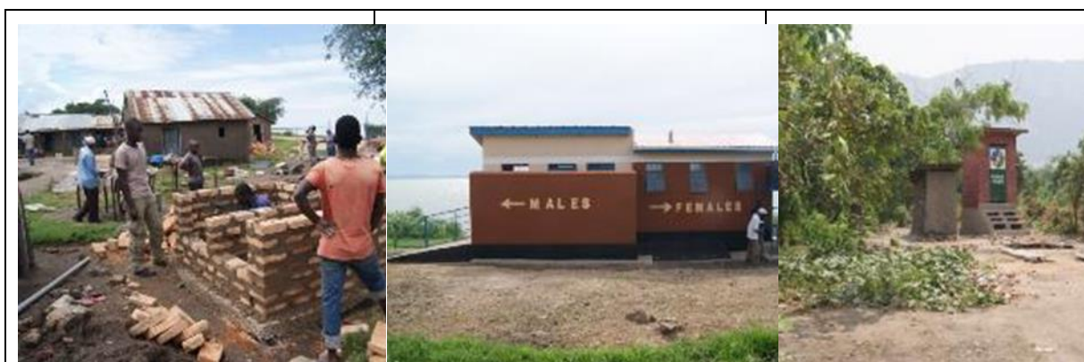
Fig. 1.17: From left to right: construction of model flower ecosan toilet, newly constructed public ecosan at landing site, flower ecosan toilet at HH
