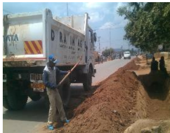
Figure 7.15 De-silting of the storm water drains
