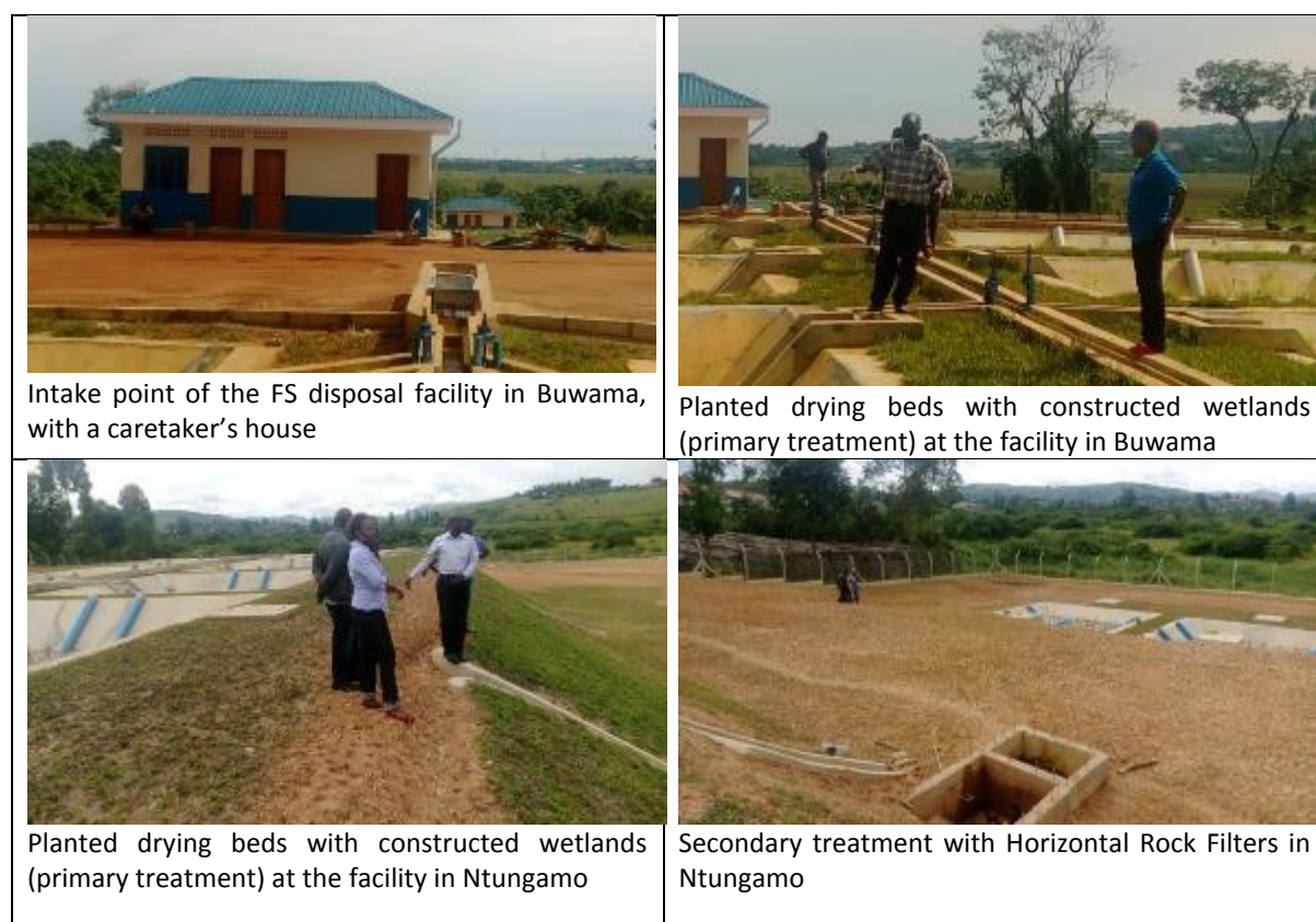
Figure 8.1 Pictures of the constructed FS disposal facilities in Buwama and Ntungamo
