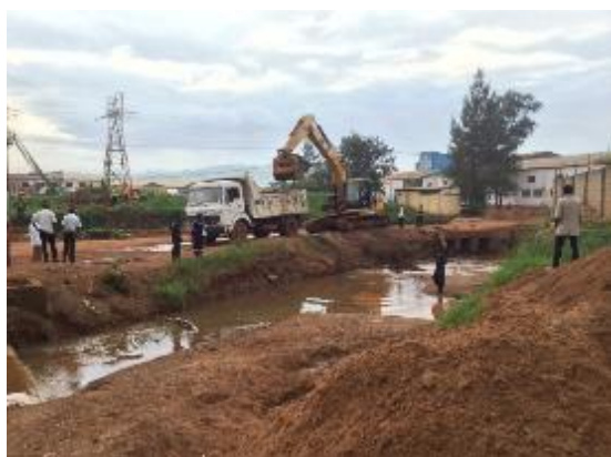
Figure 7.16 Loaders loading silt onto the truck
