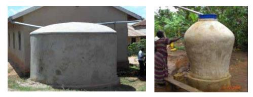
Figure 3: Ferro-cement tank (left) and cement mortar jar
