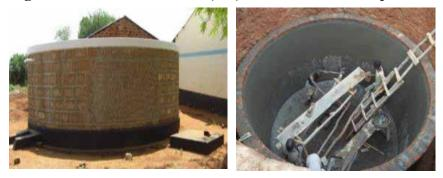
Figure 4: Above ground masonry tank (left) and below ground tank under construction
