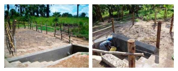
Figure 9: Medium size protected spring (left) and small size protected spring (right)
