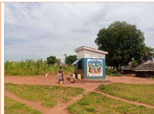
Plate 17: Existing piped water source in Pawor
